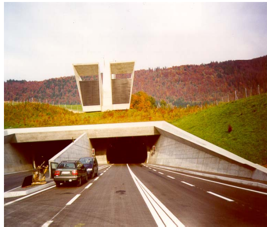
Entrance of the new Tunnel Mt. Russelin, Switzerland
