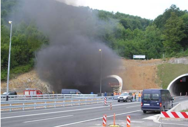
North portal of tunnel Veliki Glozac during fire test
