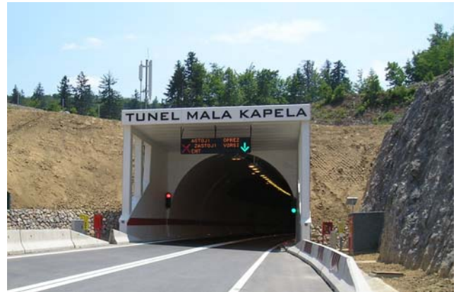
North entrance tunnel "Mala Kapela" before opening second tube
